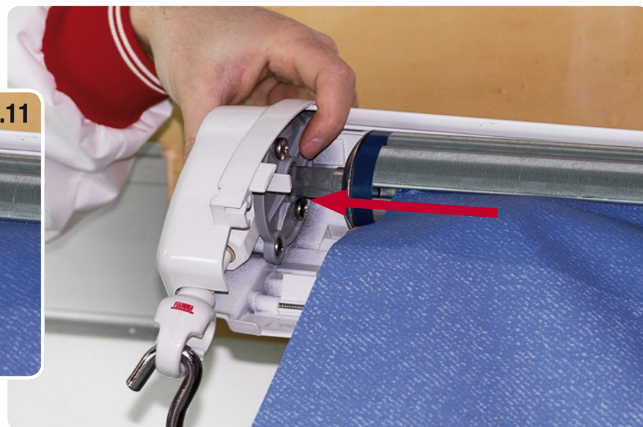
B.11 • Insert the roller tube in the left end cap.
